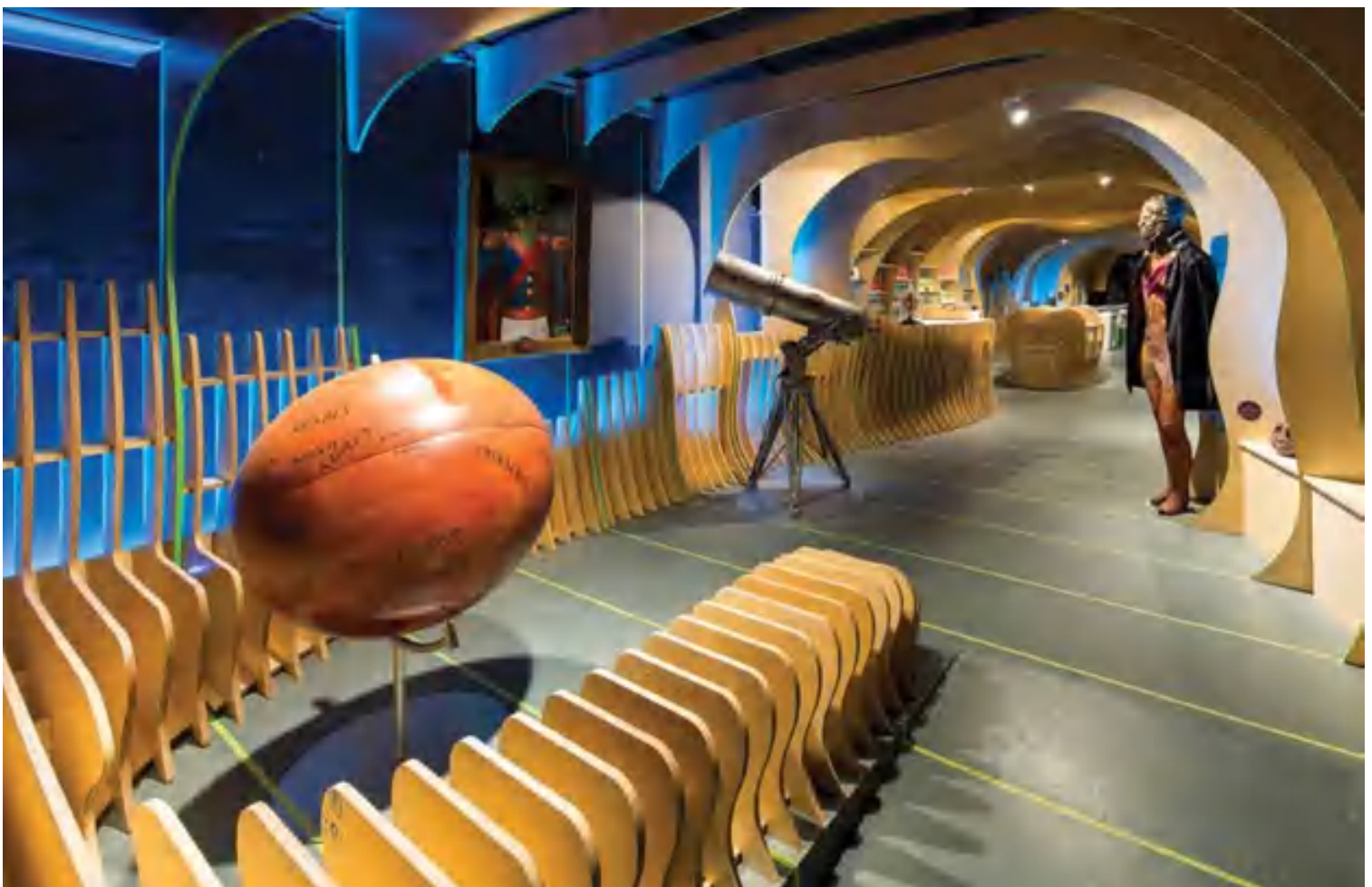
The ribbed look was created using low-grade, inexpensive plywood cut into curved shapes.
